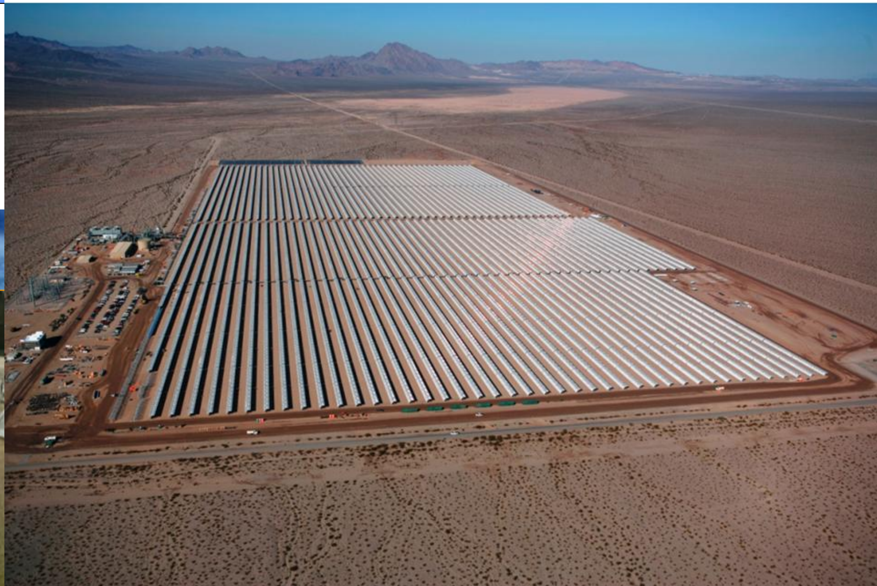
NEVADA SOLAR ONE – ACCIONA SOLAR POWER
