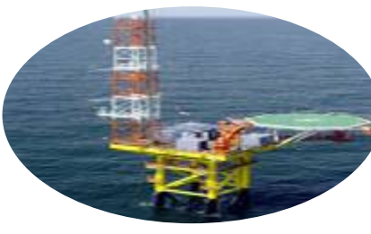
Fino Platforms Federal Ministry for the Environment, Nature conservation and Nuclear Safety (BMU)
